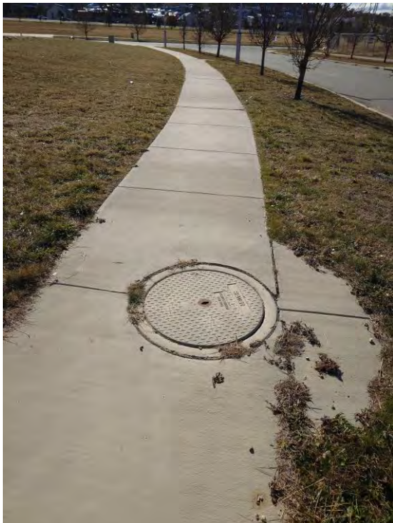
Figure 19 – Sewer Manhole in West Verge of Hoffmann Street South East of Site
