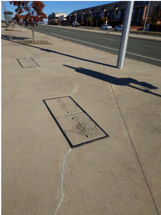
Figure 42 – NBN Pit in East Verge of Mirrabei Drive West of Site
