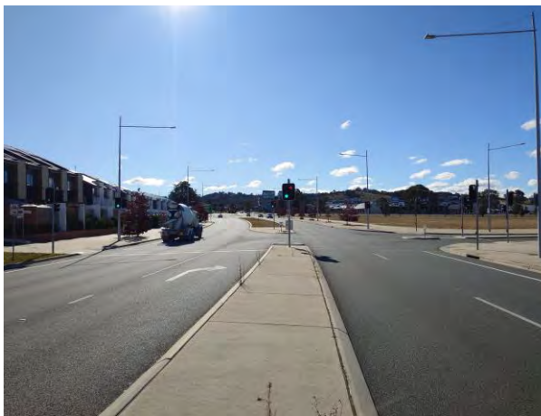
Figure 60 – Mirrabai Drive Intersection with O'Keefe Avenue Looking North
