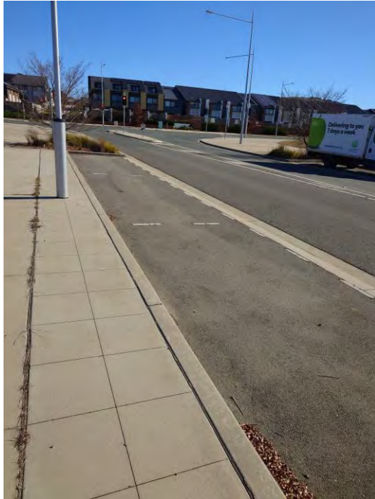
Figure 75 – On Street Car Parking on O'Keefe Avenue
