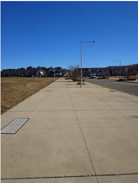
Figure 46 – TCCS Streetlights North of Subject Site
