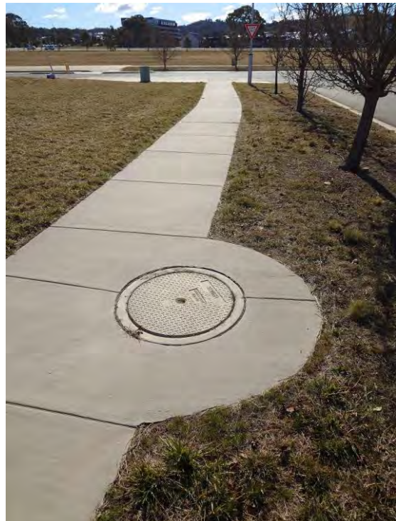
Figure 20 – Sewer Manhole in West Verge of Hoffmann Street East of Site
