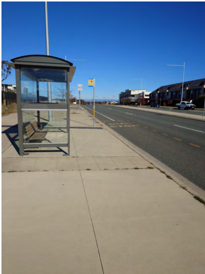
Figure 85 – Bus Stop Shelter on Mirrabiel Drive South West of the Site
