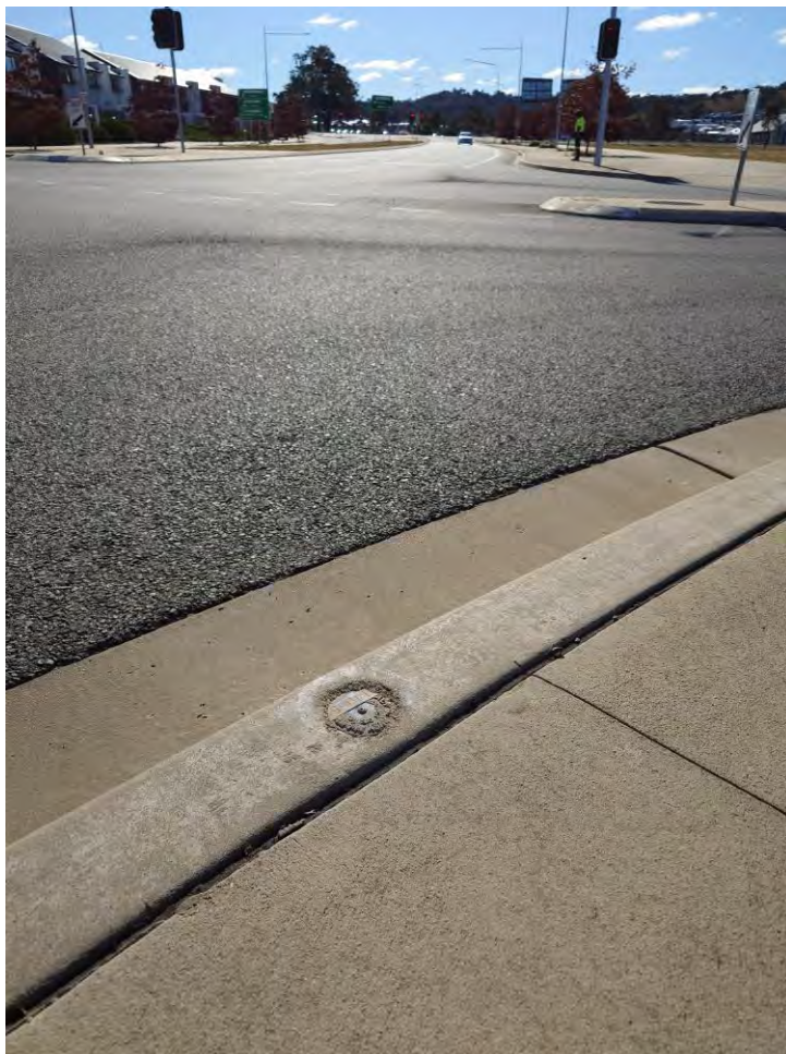
Figure 55 – Existing Kerb Survey Marker (CRM14065)
