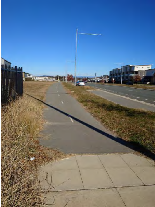
Figure 78 – Shared Path in East Verge of Mirrabai Drive
