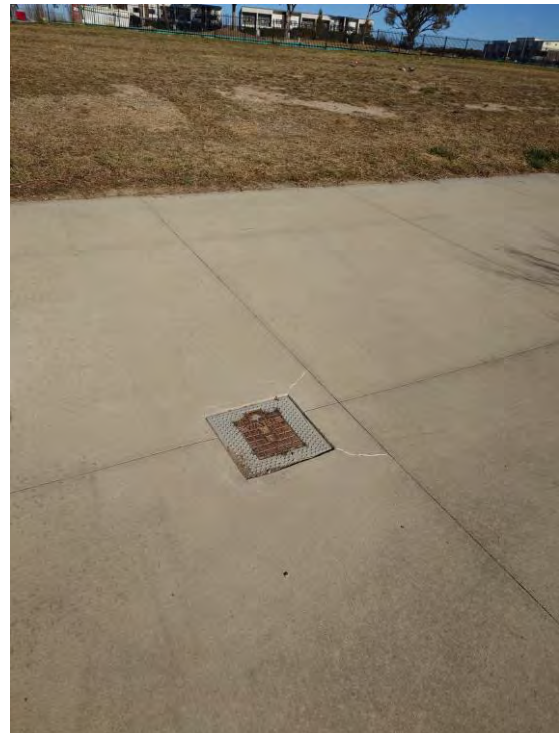
Figure 24 – Hydrant in Southern Verge of O’Keefe Avenue North of Site
