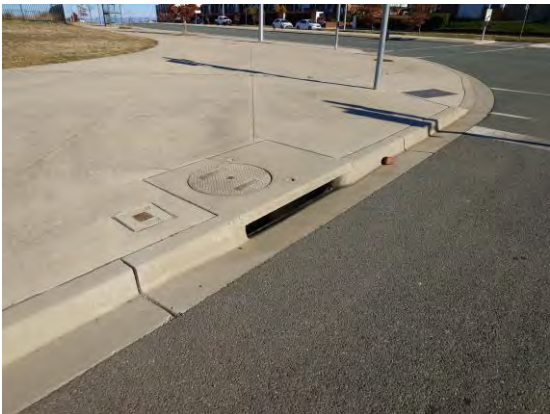
Figure 30 – Stormwater Sump at Intersection of O'Keefe Avenue and Mirrabei Drive
