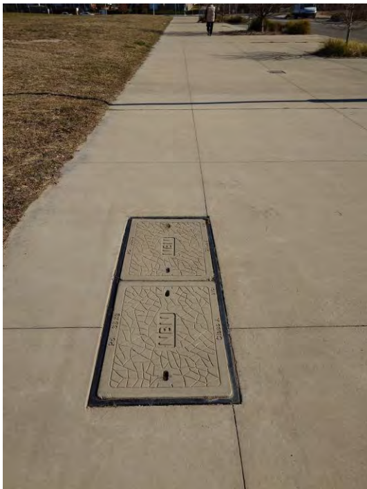
Figure 40 – NBN Pit in Southern Verge of O'Keefe Avenue North of Site
