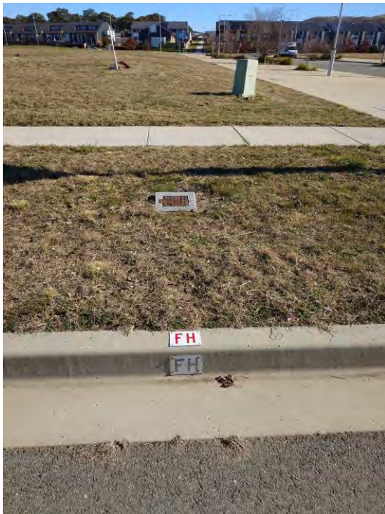
Figure 23 – Hydrant in West Verge of Hoffmann Street North East of Site
