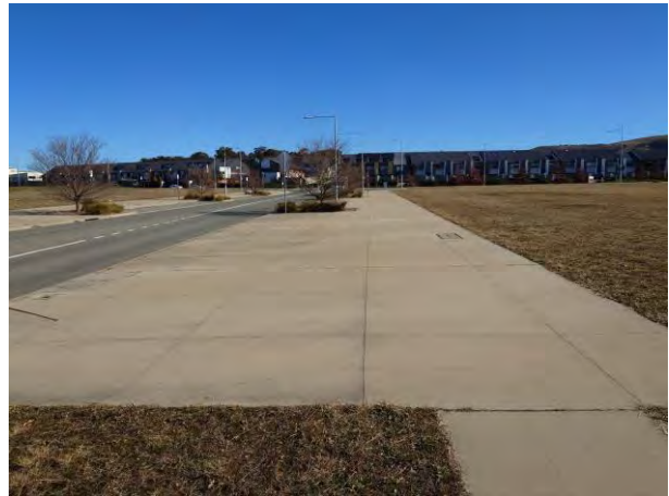
Figure 81 – Fully Paved Verge North of Site in Southern Verge of O'Keefe Avenue
