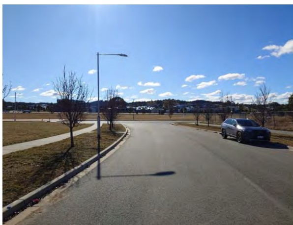
Figure 57 – Hoffmann Street East of Site Looking North
