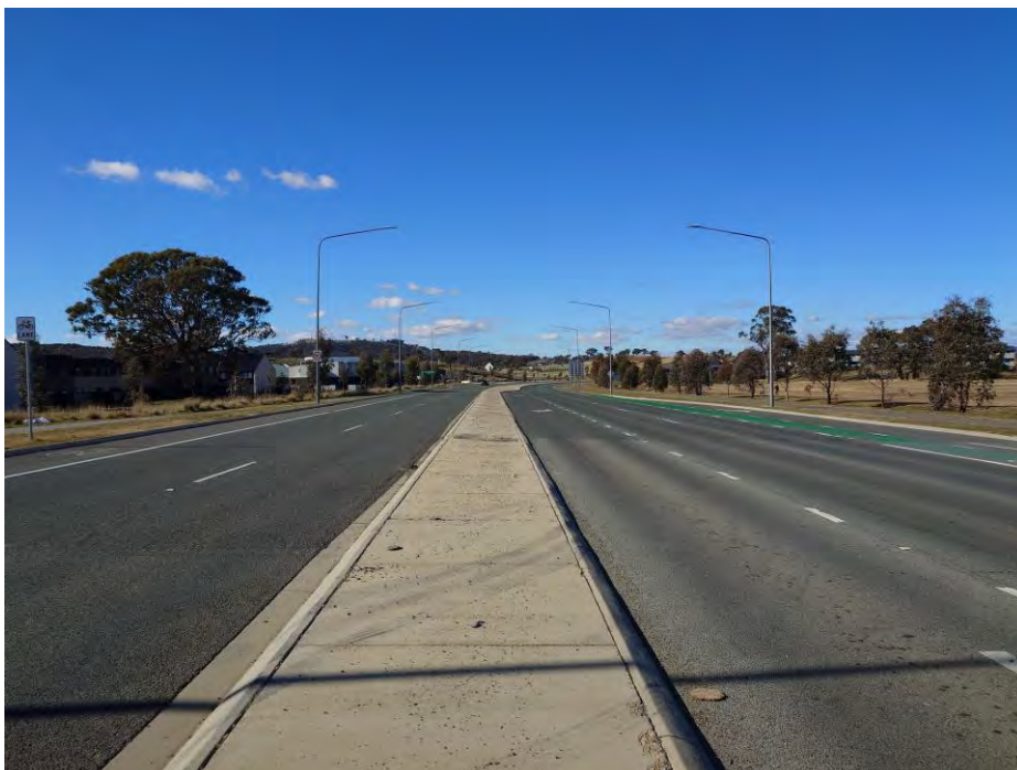
Figure 65 – General View of Horse Park Drive from Mirrabai Intersection Looking East
