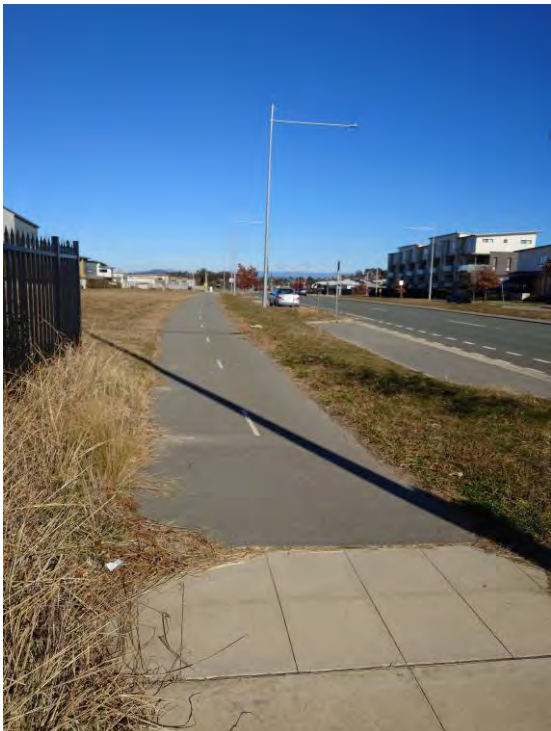
Figure 48 – TCCS Streetlights on Mirrabai Drive West of the Site
