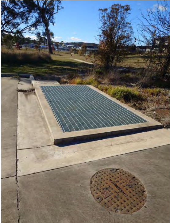
Figure 33 – Gross Pollutant Trap North East of the Site in Open Space
