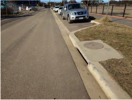
Figure 28 – Stormwater Sump at Junction of DN525 from Kate Crace Street and DN300 from Camilleri Way to a DN600 Pipe
