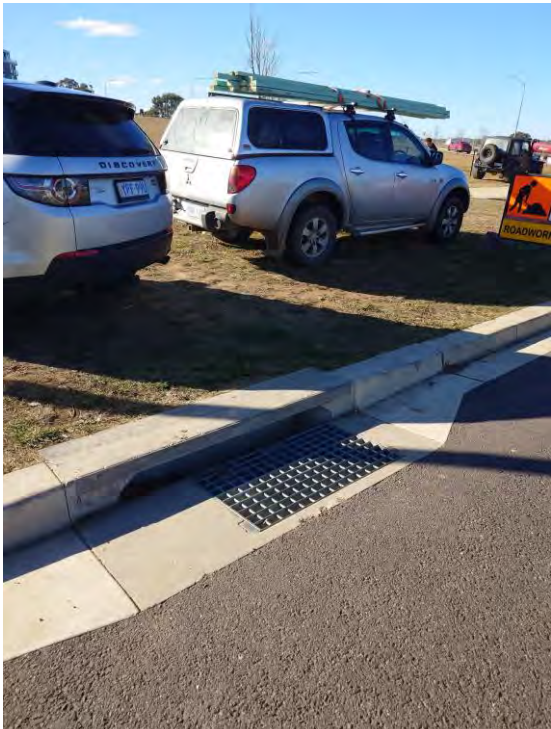
Figure 31 – Stormwater Sump South of Site
