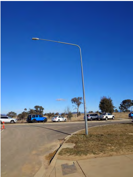
Figure 44 – Streetlight in Kate Crace Street South East of Subject Site
