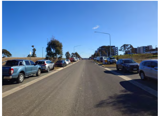
Figure 68 – Camilleri Way On Street Car Parking
