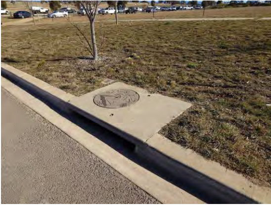
Figure 29 – Existing Stormwater Sump in Kate Crace Street East of Site
