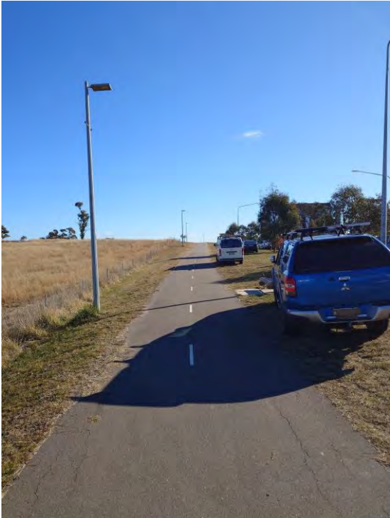
Figure 43 – Streetlights along Shared Path South of the Site
