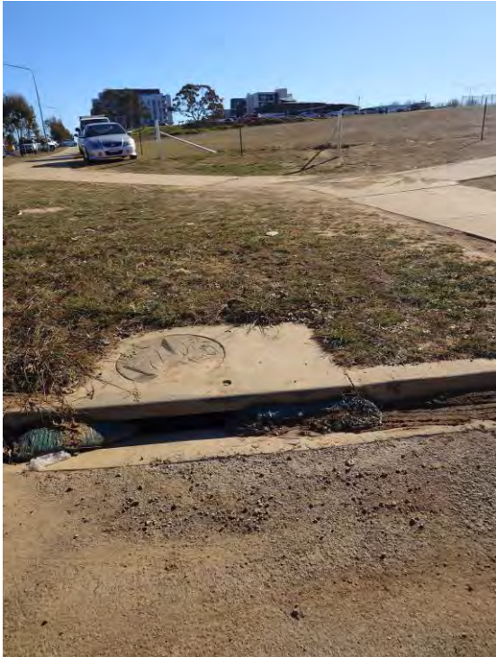
Figure 30 – Stormwater Sump South East of Site
