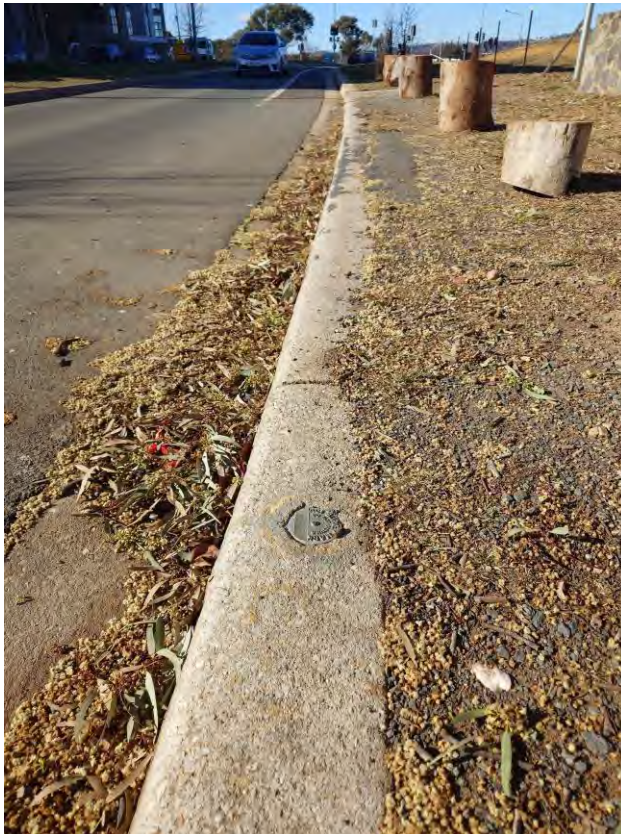
Figure 50 – Kerb Survey Marker on The Valley Avenue (CRM11556)
