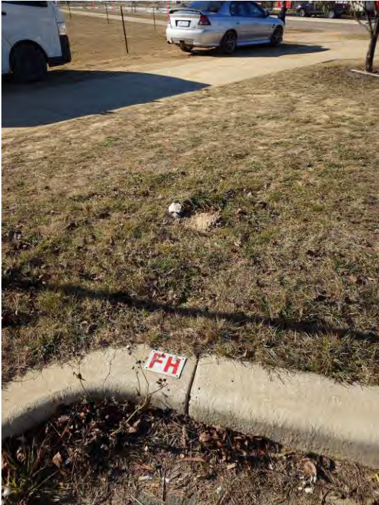
Figure 21 – Existing Hydrant Directly South of Site
