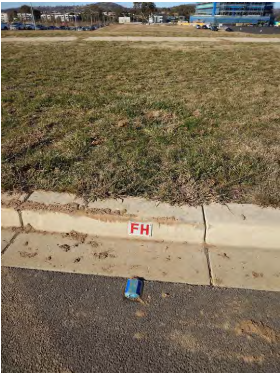
Figure 22 – Existing Hydrant North East of Site
