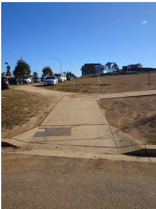
Figure 73 – Footpath Connections Looking Toward South East Corner of Site
