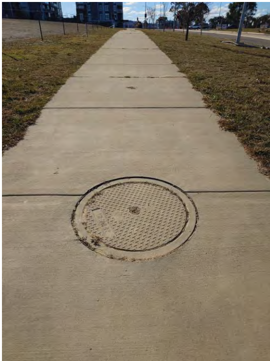
Figure 18 – Sewer Manhole North East of Site
