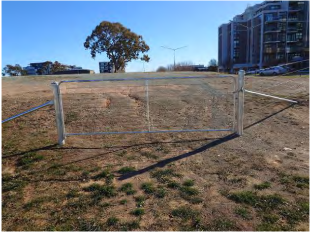
Figure 55 – Access gate to Block 3 Section 235
