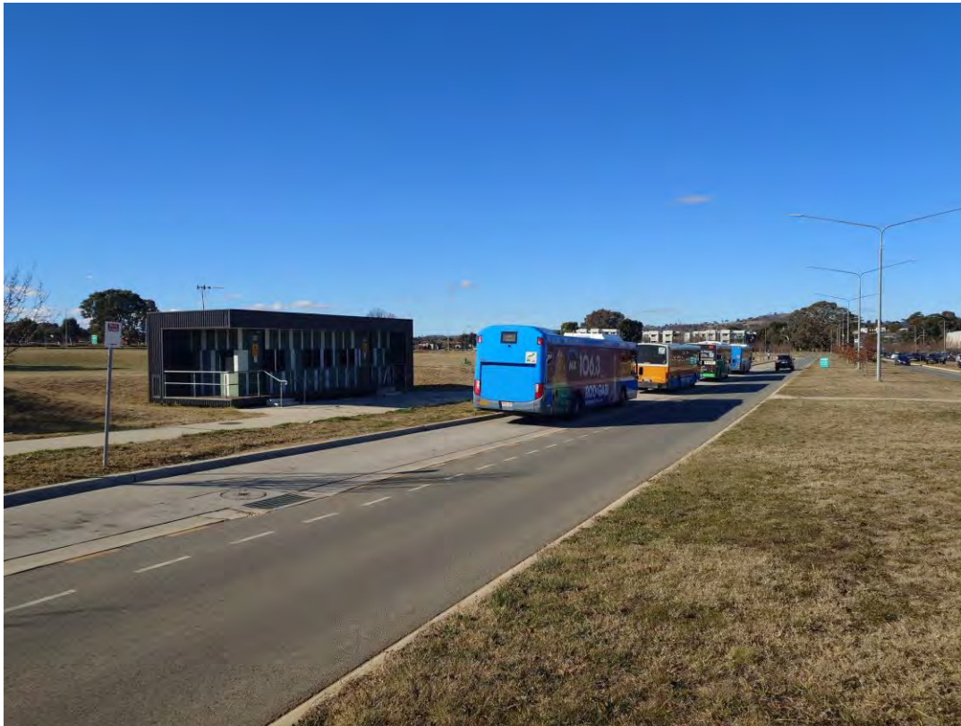
Figure 76 – Bus Rest and Stop Shelter on The Valley Avenue North East of the Subject Site
