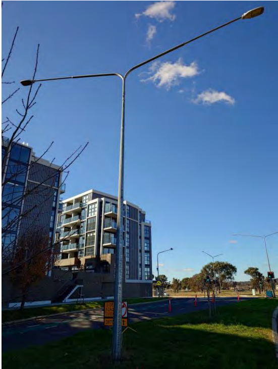
Figure 45 – Dual Mast Streetlights in The Valley Avenue Central Median
