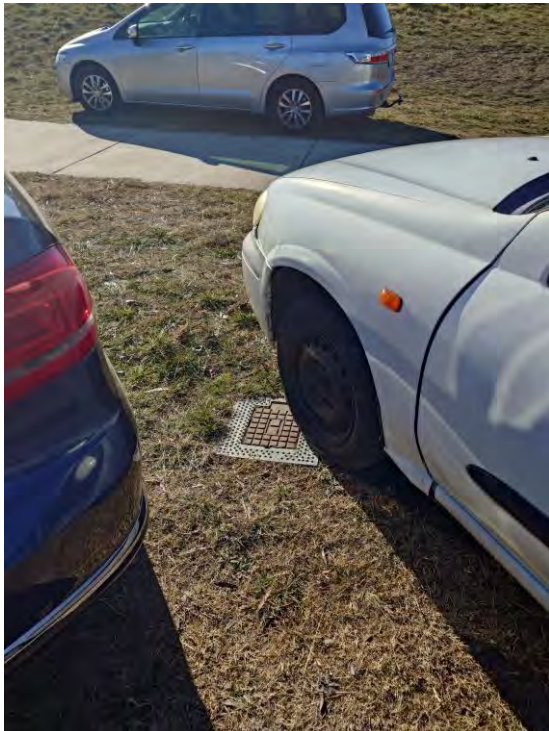
Figure 25 – Existing Hydrant South West of Site
