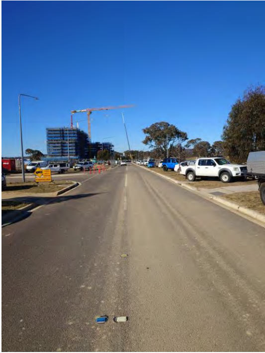
Figure 56 – Camilleri Way Looking East
