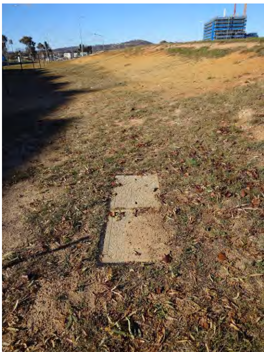
Figure 35 – Telstra Pit over Telstra Service in The Valley Avenue
